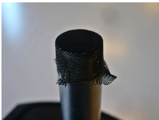
Strainer blocked by soot
